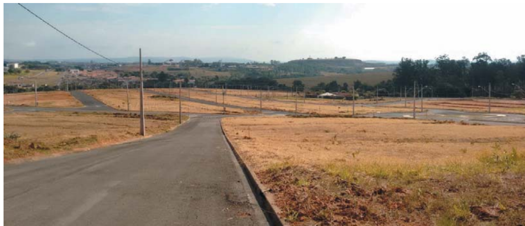
Vista parcial do loteamento Village Paraíso
